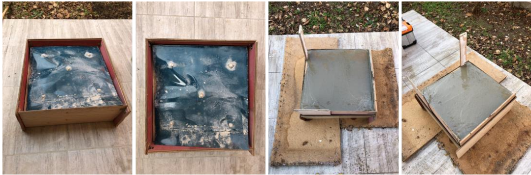
Figure 29: Horizontal concrete component production with recursive and re-usable formwork. Framed with flat wooden supports for a concrete pour, developed and photographed by the author.
