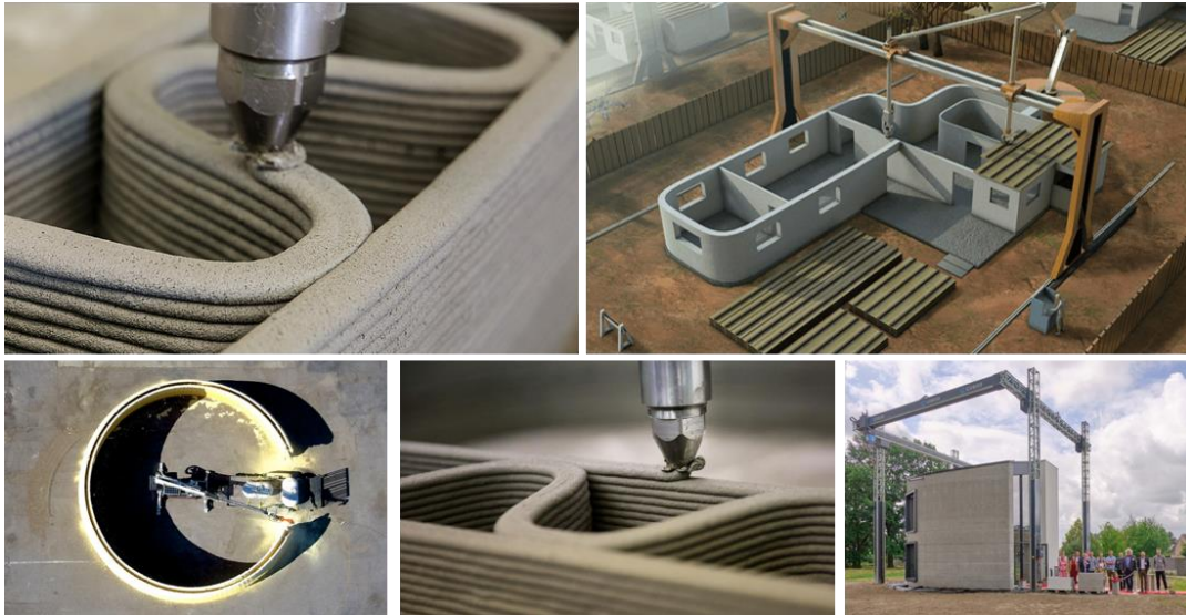
Figure 9: Additive concrete manufacturing process photographs.
